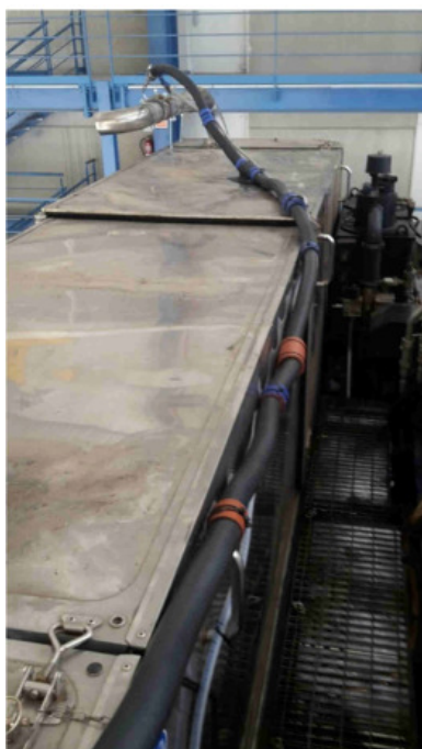
Figure 42. Bundle of heated gas sampling, pressure and temperature lines
