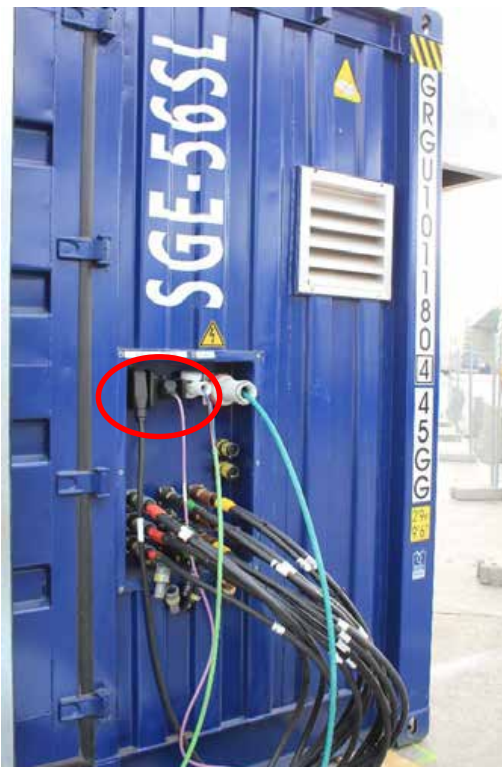
Figura 104. Control signal between the engine container and the ship (through the shore transformer).
