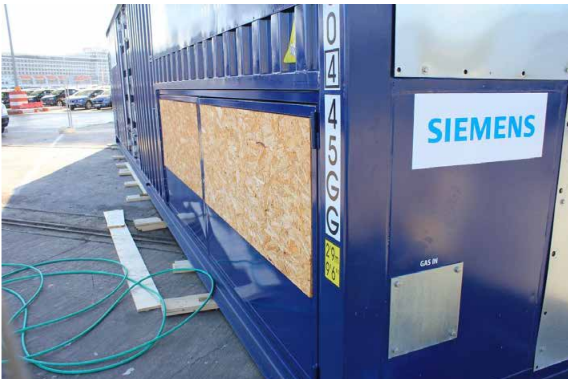
Figura 131. Removing protection plates for transport. Protection plates for the gas train or ventilation area.
