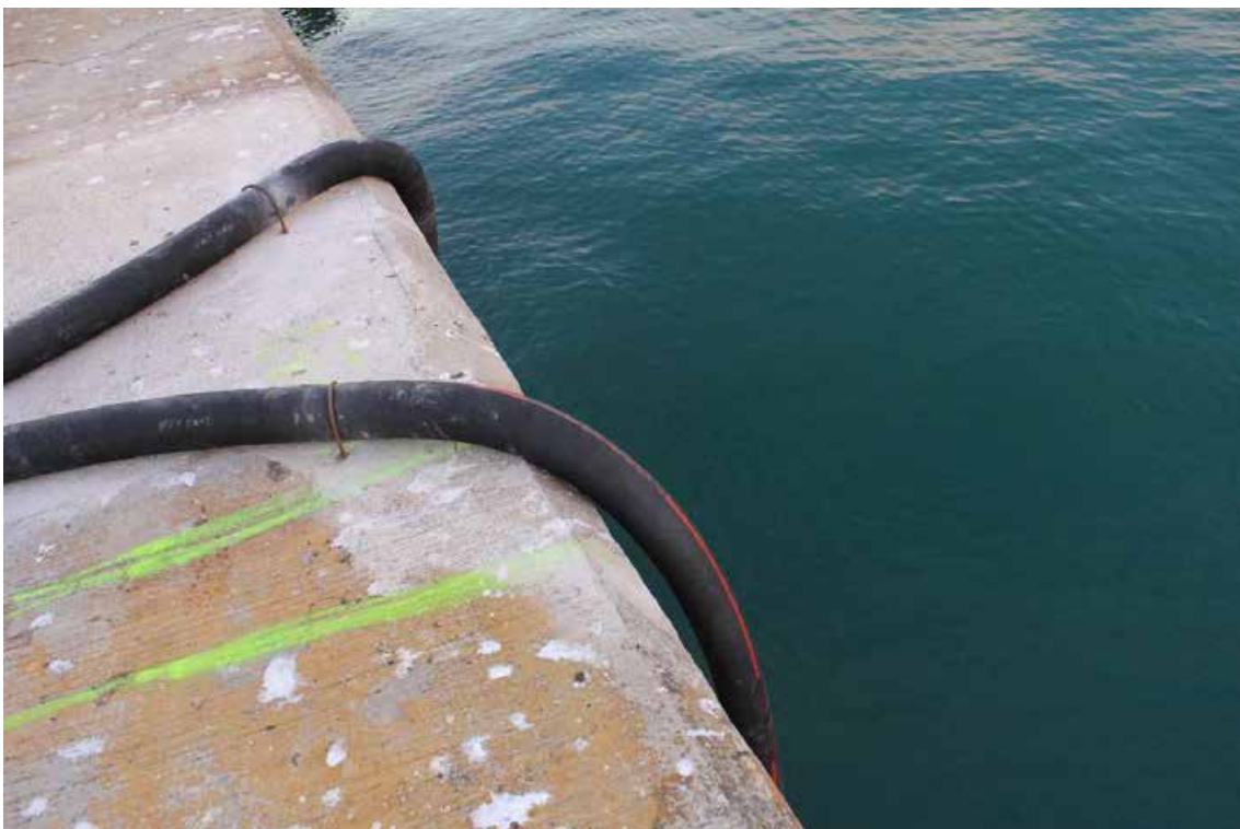
Figura 60. Installing the ND100 pipes of the secondary refrigeration circuit.
