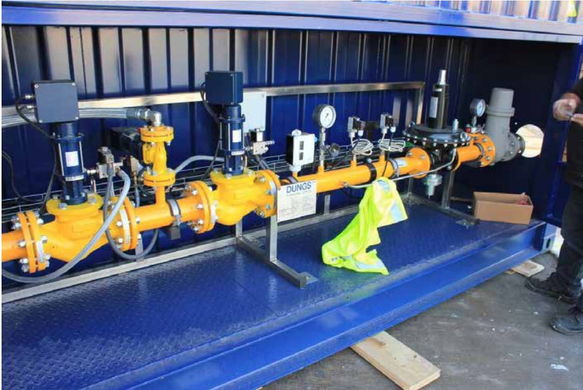
Figura 70. Gas train of the engine container.
