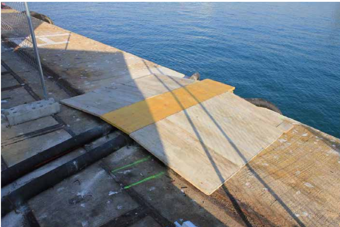
Figura 68. Protection to allow pedestrians to walk above the pipes.
