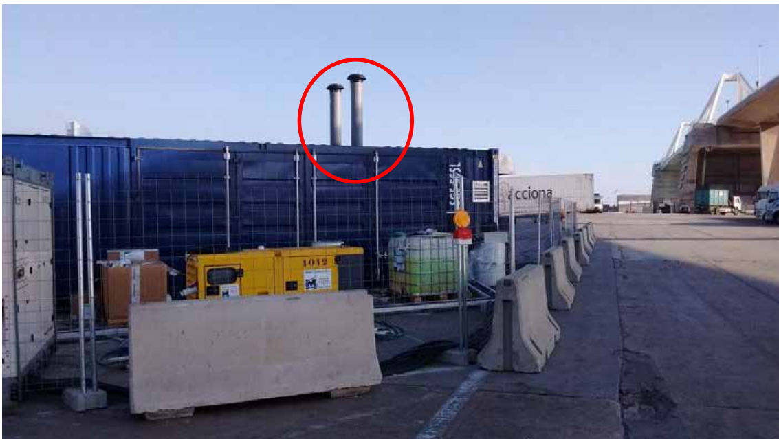
Figura 136. Installing the air intake pipes to the engine.
