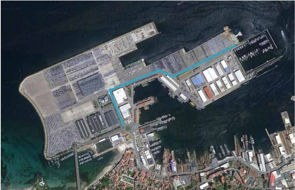
Figure 27: Detail of the access to the Ro-Ro Terminal. In blue, entrance and exit route.
