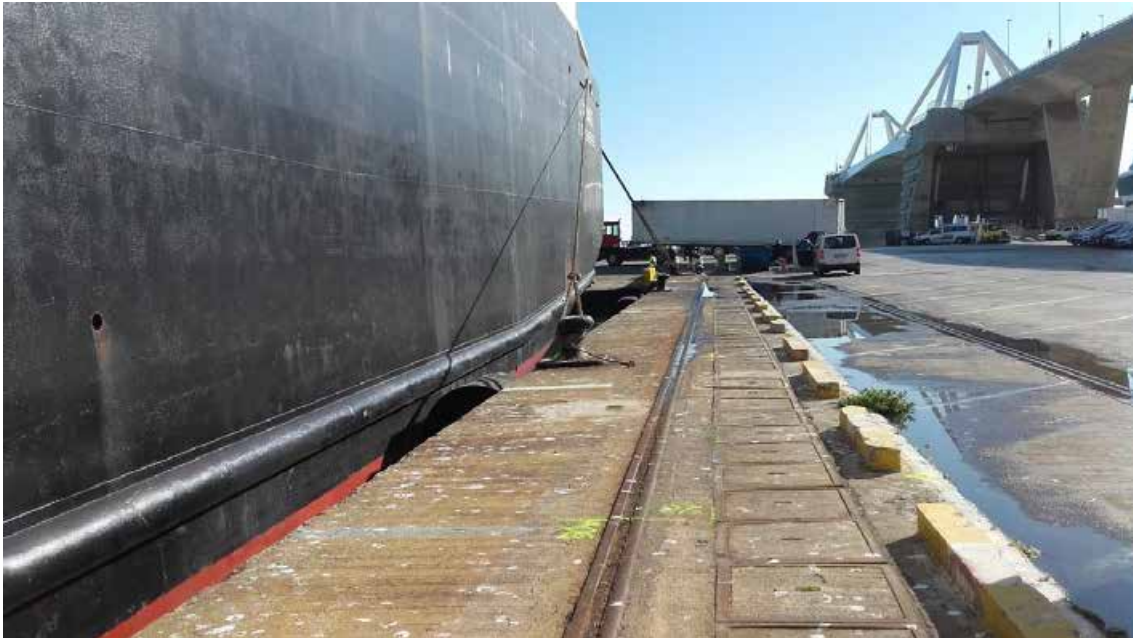
Figura 8. General view of the Ponent wharf with the L'Audace docked.
