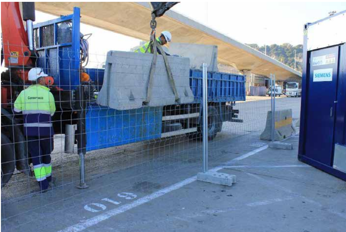
Figura 27. Installation of the New Jersey-type fence and Rivisa fence.
