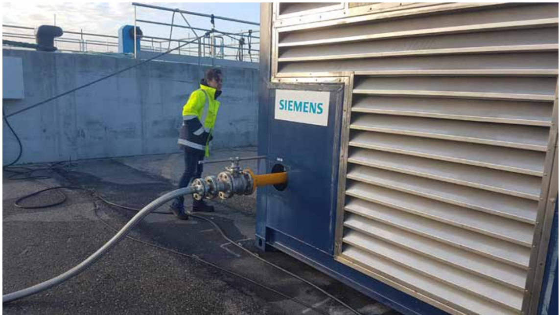
Fig.11. Connection of the gas hose
