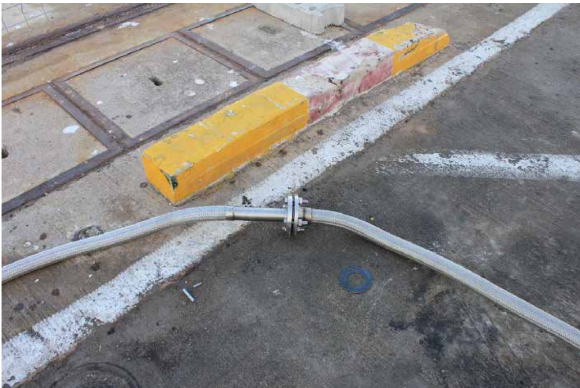
Figura 76. Flange for joining the gas hoses.
