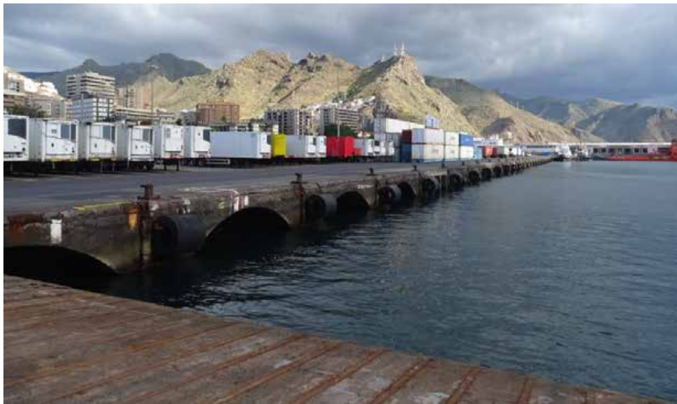
Figure 5. General view. Muelle de Ribera .
