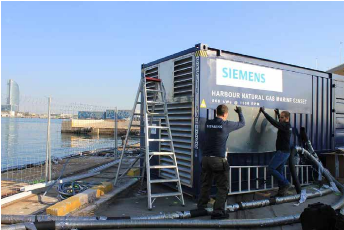
Figura 130. Removing protection plates for transport.
