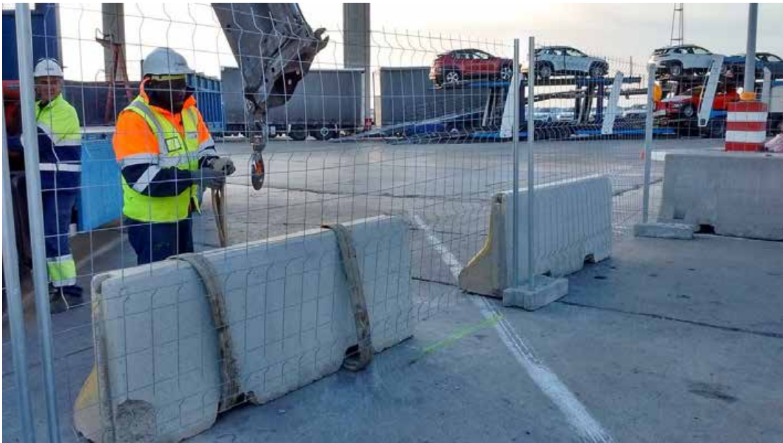
Figura 26. Installation of the New Jersey-type fence and Rivisa fence.
