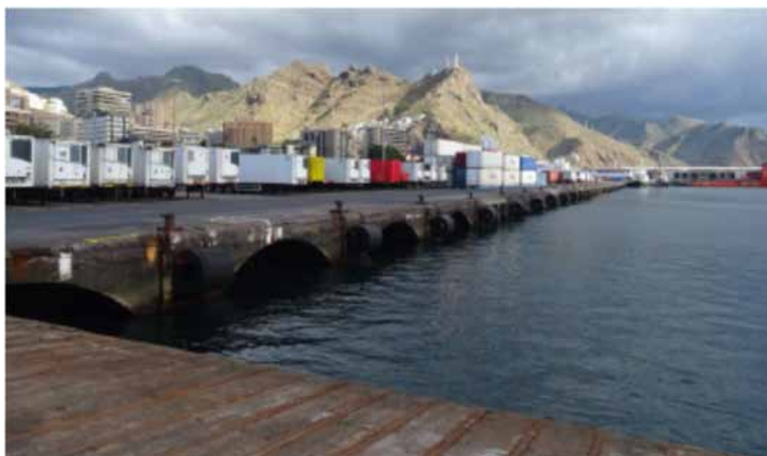
Figure 35: General view of La Ribera Quay.
