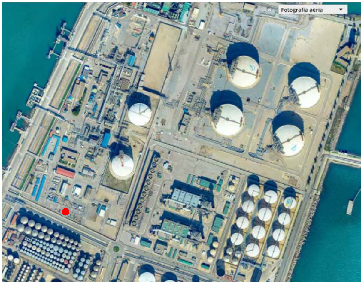
Figura 4. Equipment storage area at the Enagás plant.
