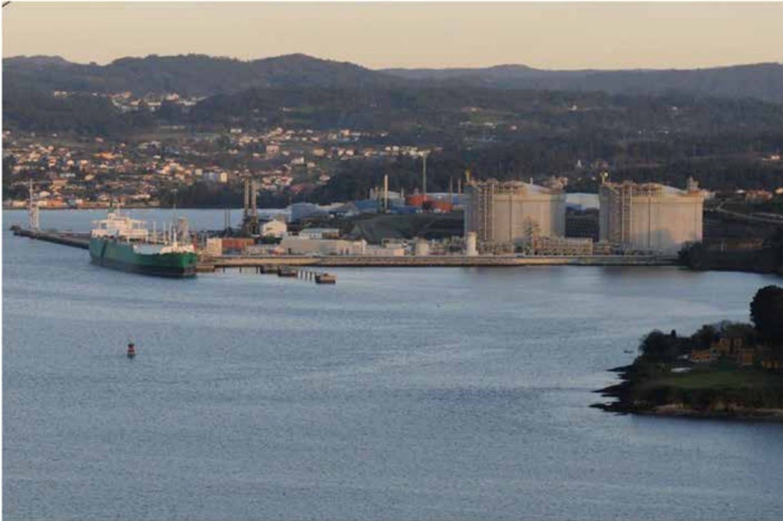
Figure 25: View of the Reganosa regasification plant (source: Reganosa)
