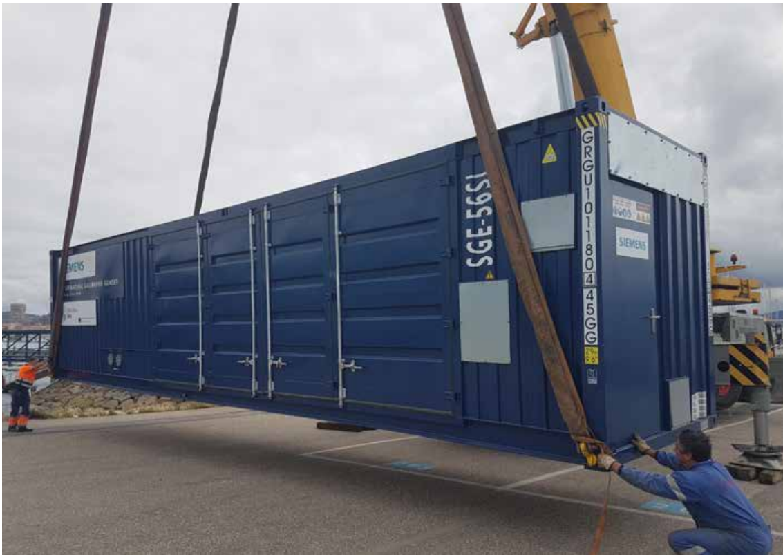
Fig.5. Unloading and placement of the equipment
