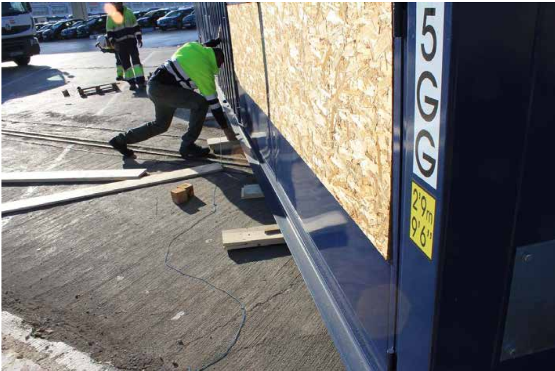
Figura 16. Placing wooden planks to correctly support the generator engine.
