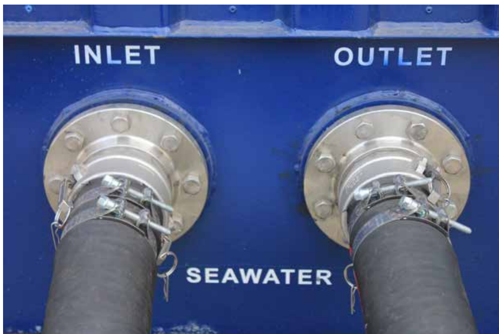
Figure 31. Installation of the DN100 pipes of the secondary refrigeration circuit.
