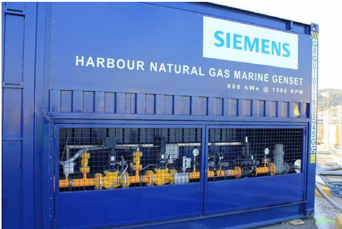
Figura 132. Removing protection plates for transport. Gas train protection plates.
