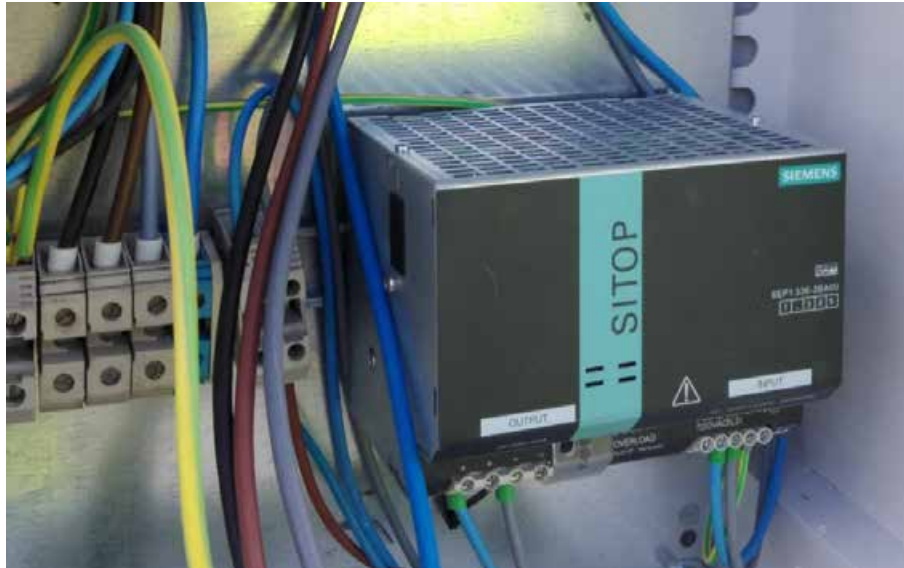
Figure 22. 24V and 20A power supply, SITOP 6EP1366-3BA00.
