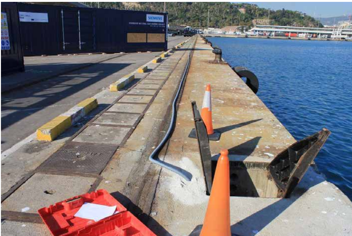
Figura 52. Installation work for the 230v connection for the tank container.
