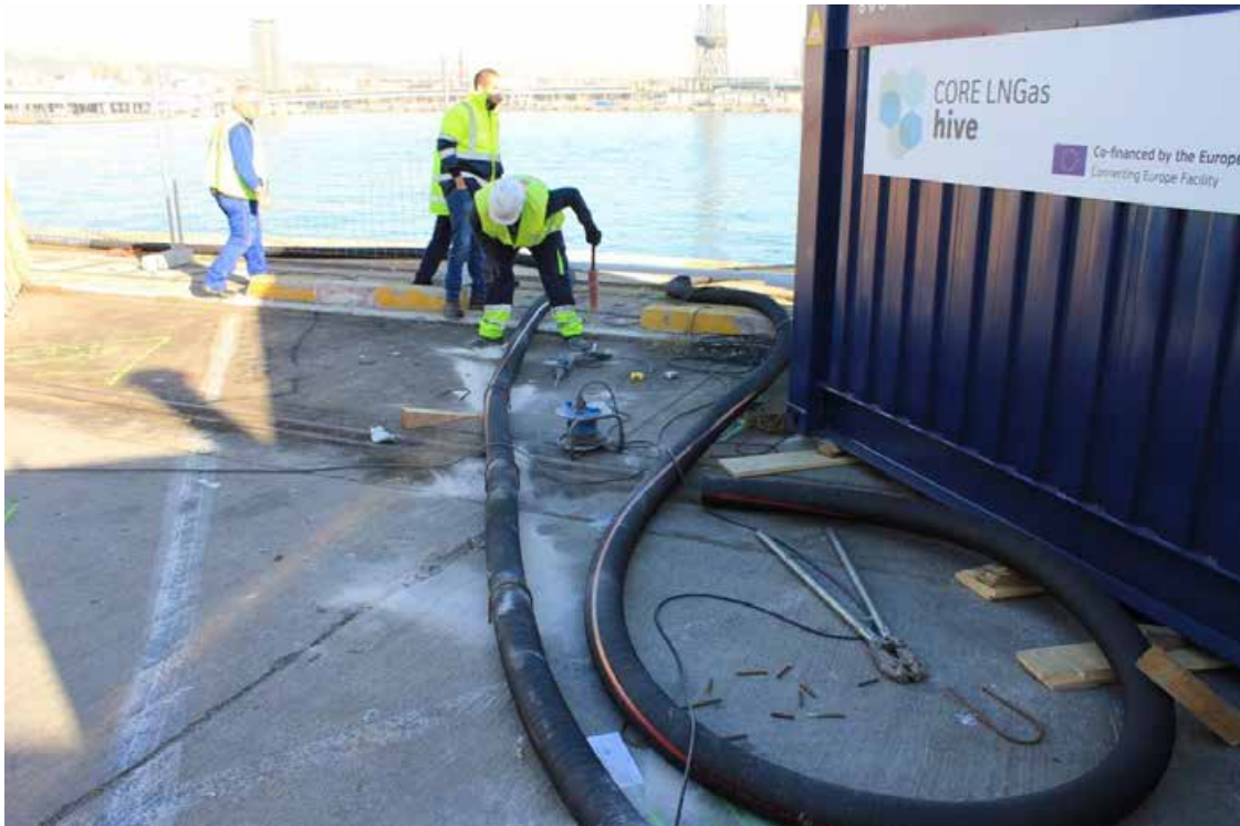
Figura 57. Installing the ND100 pipes of the secondary refrigeration circuit.
