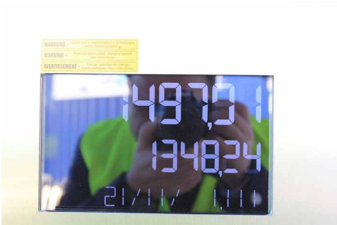
Figura 129. Tank control panel. Quantity supplied.
