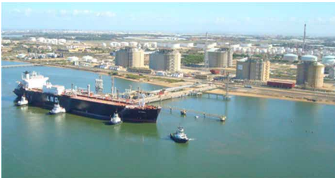
Figure 33: View of the Huelva regasification plant (source: Enagas)
