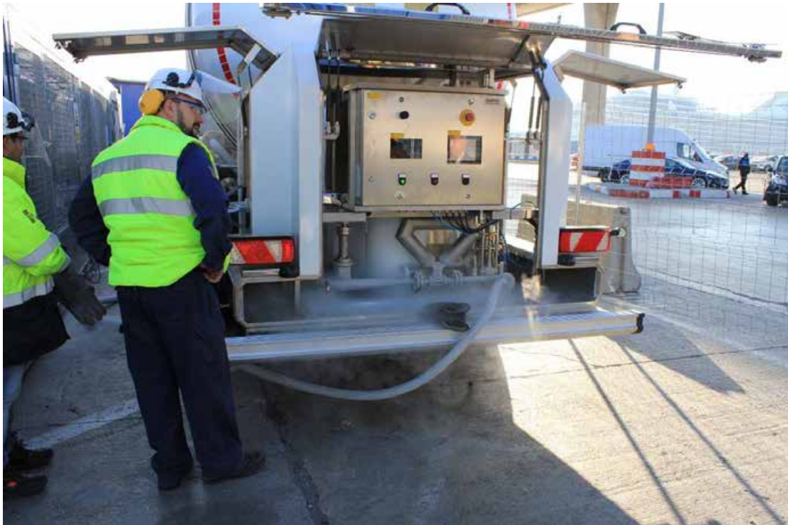
Figura 121. Tank control system. The white haze visible is due to the condensation of humidity due to the cooling of the pipes by the passage of LNG to -145^{\circ}\text{C} of temperature.
