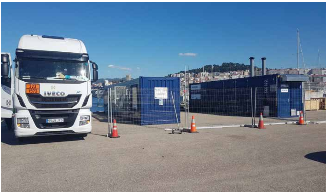
Fig.7. Fenced operation area
