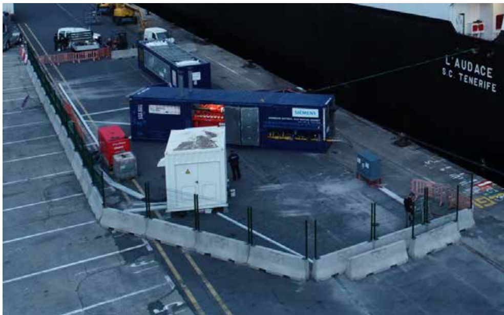
Figure 12. Installation of the New Jersey type and Rivisa fence.
