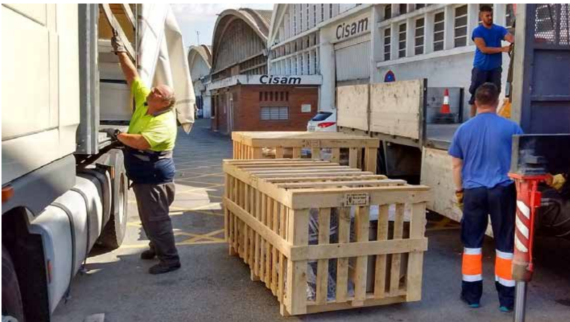
Figura 21. Unloading Guascor-Siemens equipment and materials on Sant Bertran (17 June).
