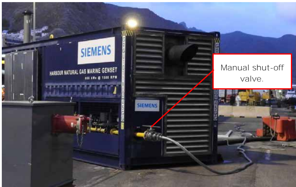
Figure 34. Gas inlet to the gas train of the engine container. Manual shut-off valve and reducer to gas hose.
