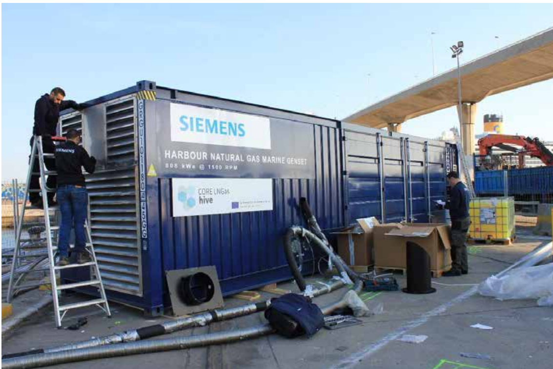
Figura 134. Removing the exhaust cover.
