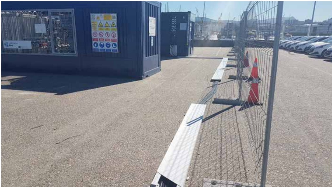
Fig.12. Power cable from the generator motor to the ship
