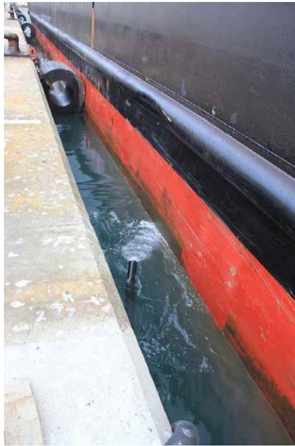
Figura 69. Sea water circuit outlet pipe, with some movement to dilute the hot water.
