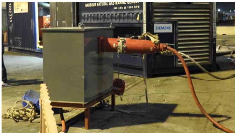
Figure 44. Connection between Monaguillo and the ship's cable.
