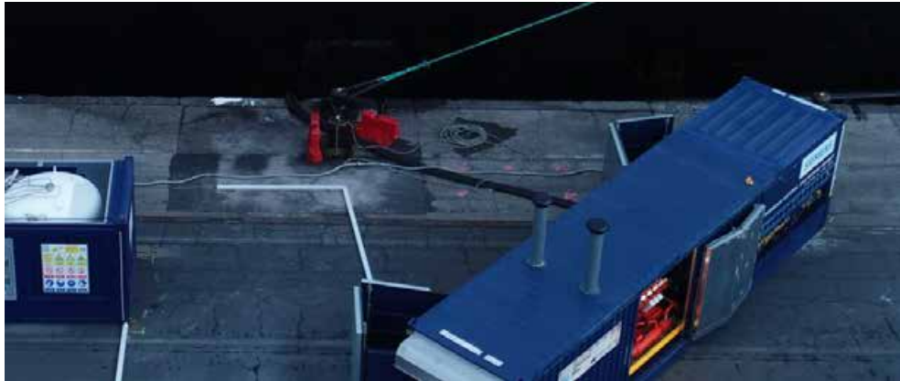
Figure 30. Installation of the DN100 pipes of the secondary refrigeration circuit.
