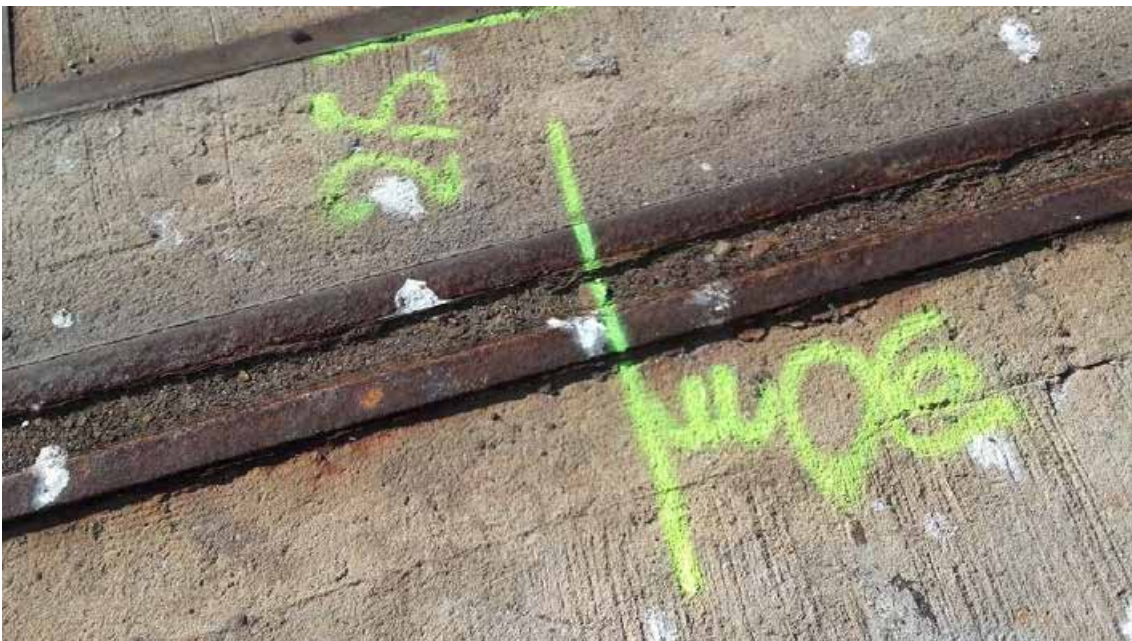
Figura 10. Marking the position of the engine container (Guascor-Siemens).
