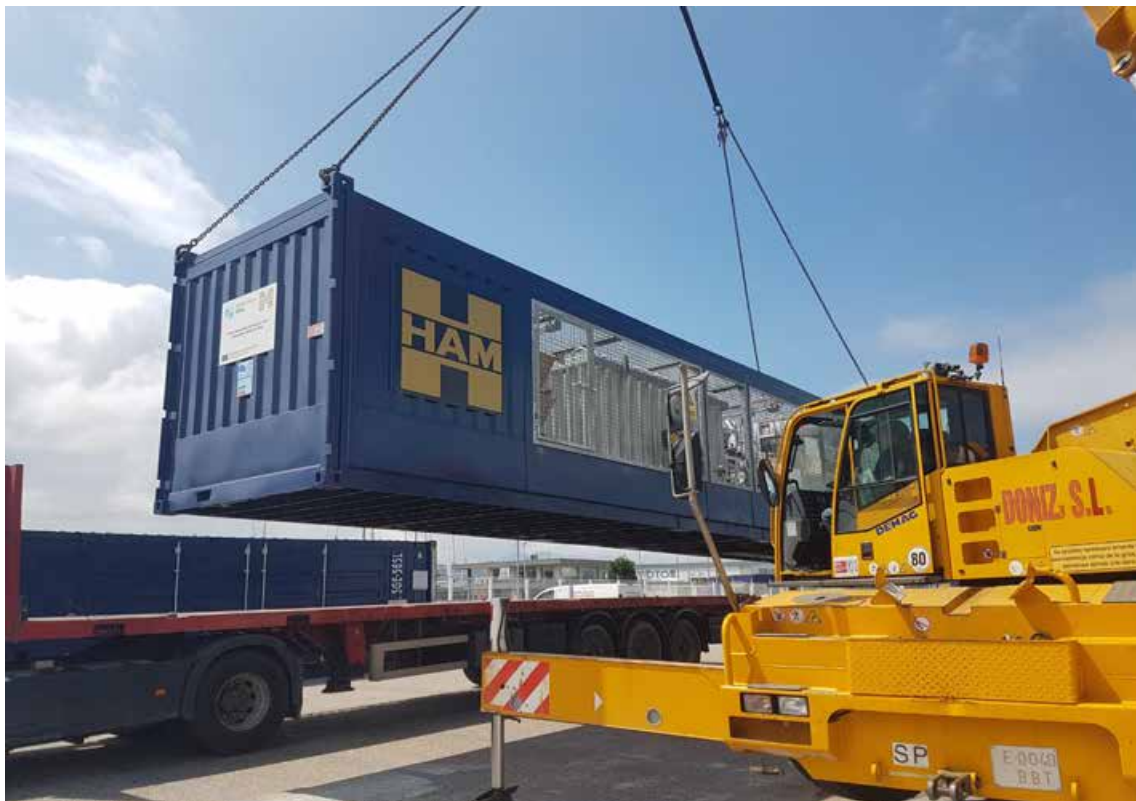
Fig.6. Unloading and placement of the equipment.
