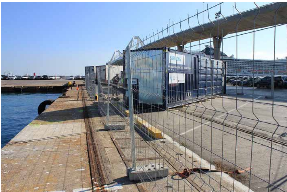
Figura 28. Installation of the New Jersey-type fence and Rivisa fence.
