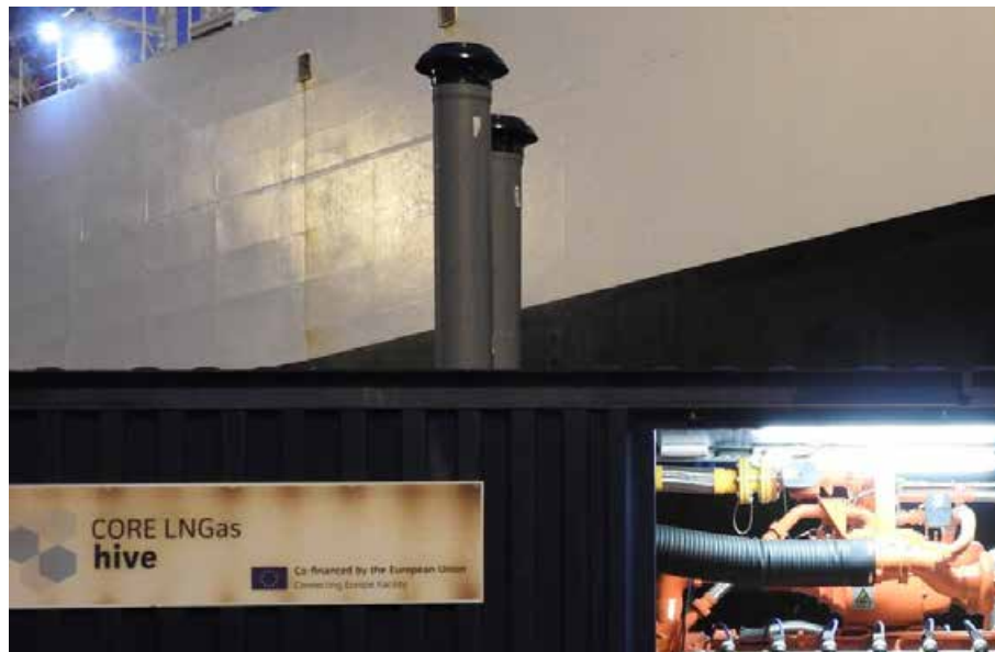
Figure 56. Installing the air intake pipes on the deck.
