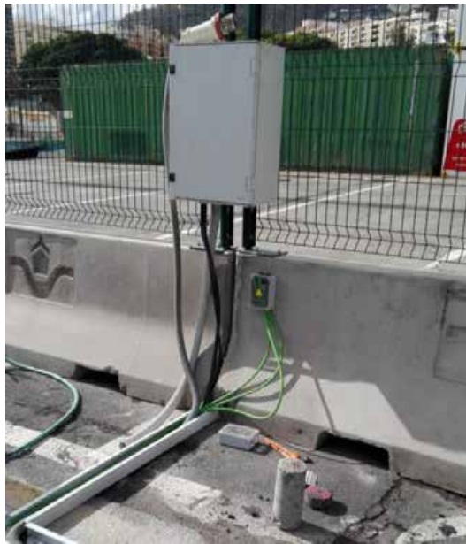
Figure 27. Installation for the 230 V connection for the tank container. Box.
