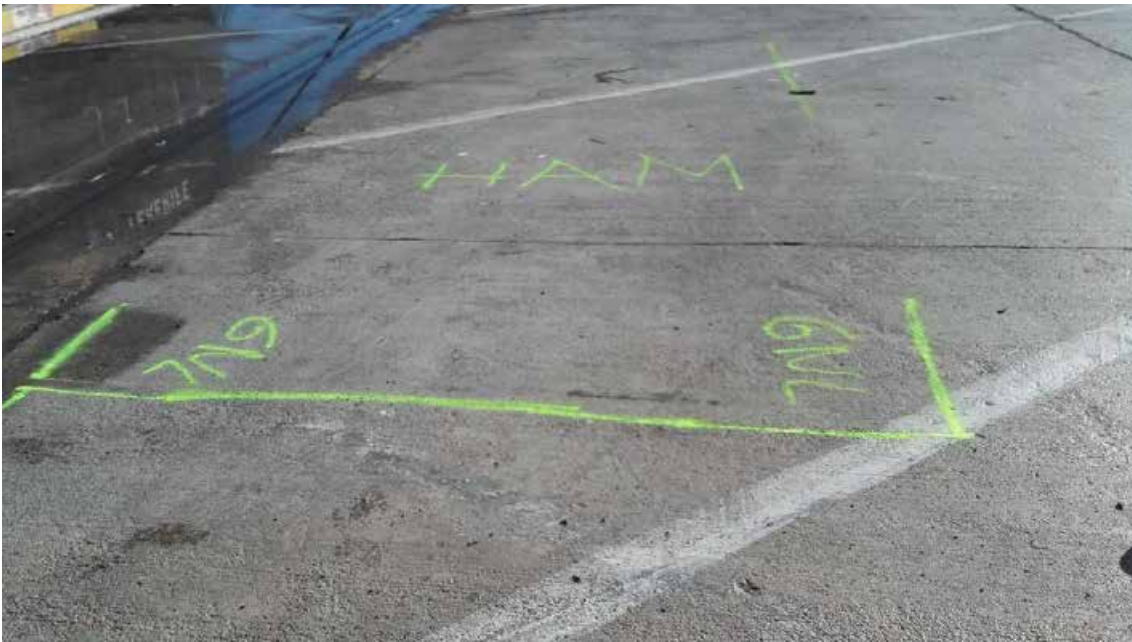
Figura 9. Marking the position of the container of the LNG tanks (HAM).
