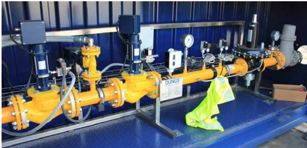
Figure 33. Gas train of the engine container.
