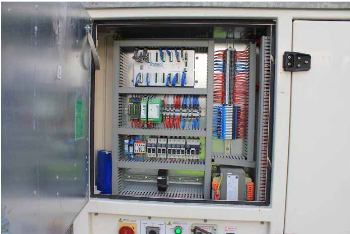
Figura 144. Resistive load bank.
