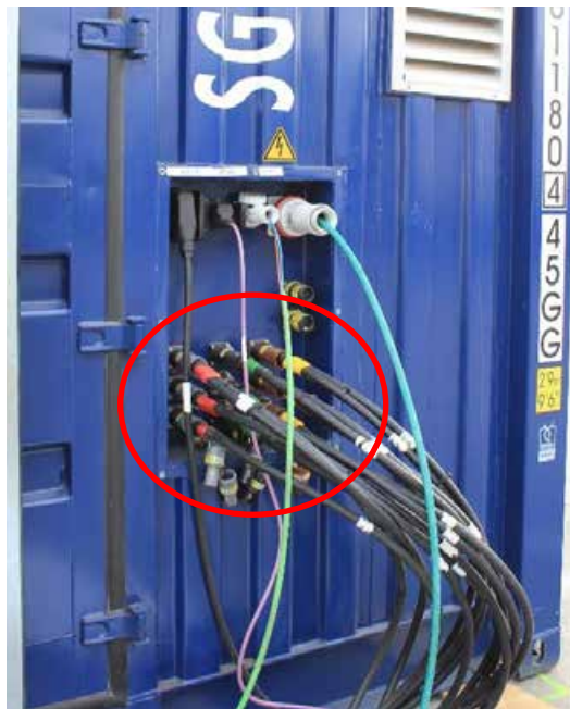
Figure 38. Motor voltage output at 400 Vac.
