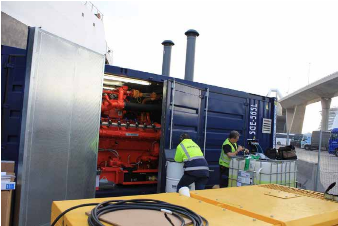
Figura 147. Engine carburetion adjustment.
