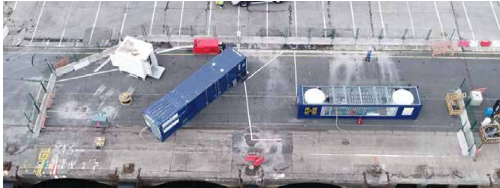
Figure 11. Installation of the New Jersey type and Rivisa fence.
