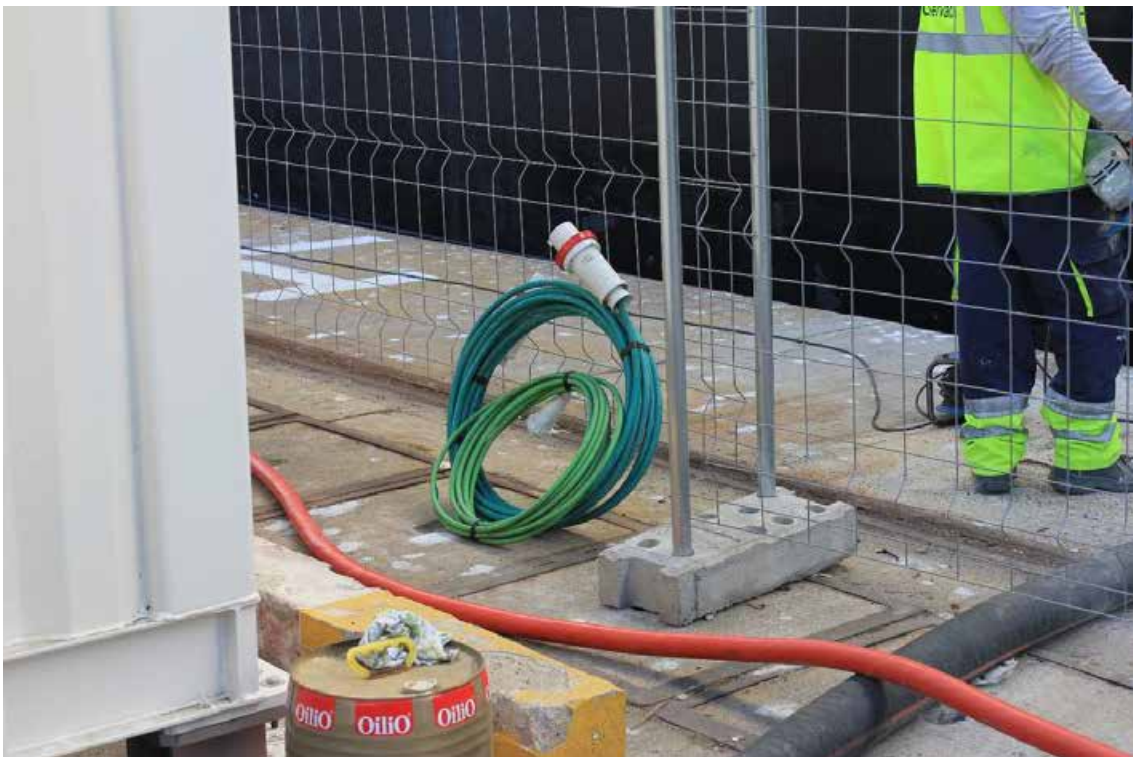
Figura 43. Cables with Pratika 81683 and Pratika 82977 connectors.
