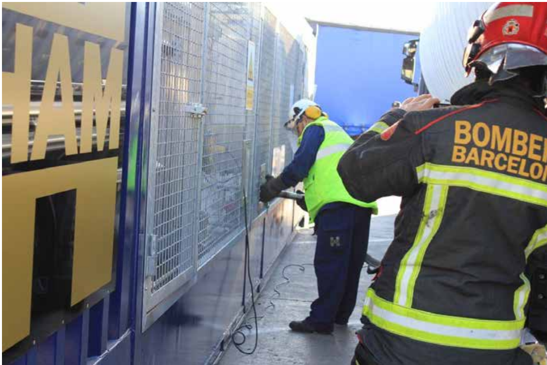
Figura 119. Connection of the earthing clamp (cable) and connection of the LNG hose to the container inlet valve (from here it is sent to one or another tank, by shower or by sump).
