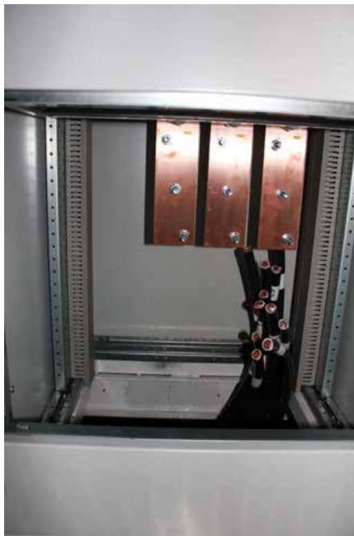
Figura 88. Earth transformer. Three-pole busbar cell for connecting the 400v wiring from the engine.
