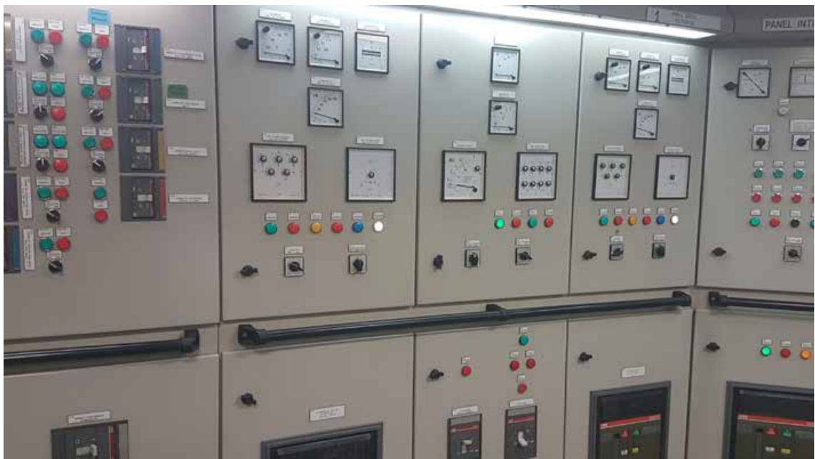
Fig.19. Test on October 17, inside the ship
