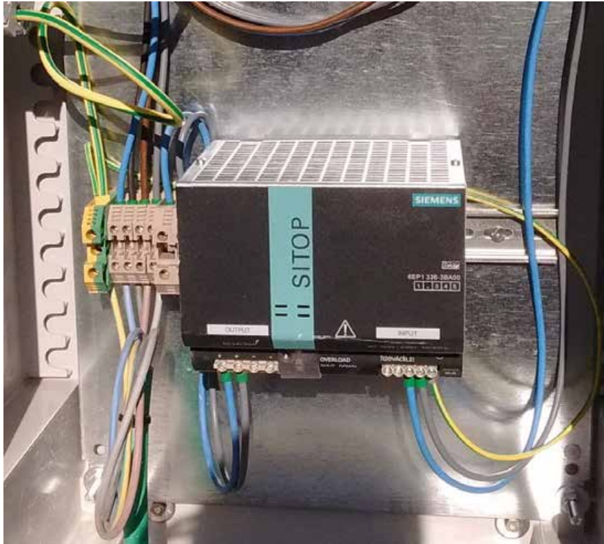
Figura 48. SITOP 6EP1366-3BA00 24v, 20A power supply.
