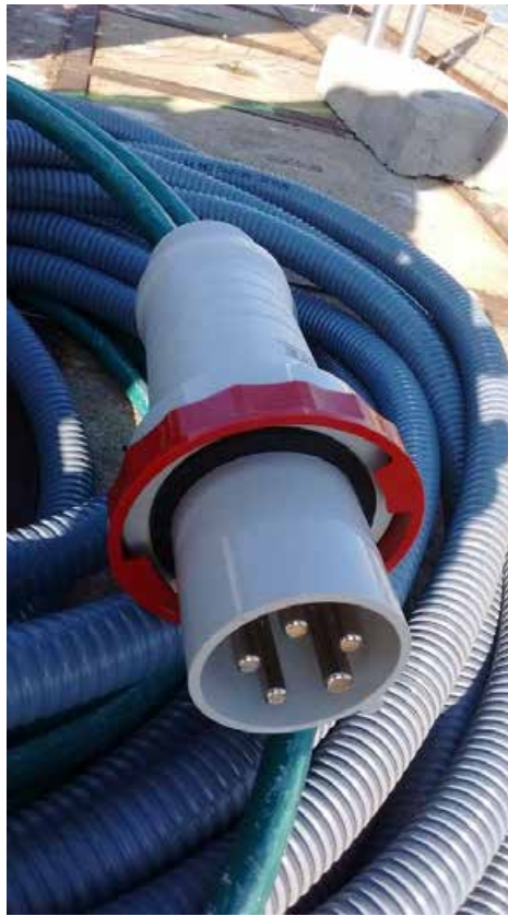
Figura 40. Pratika 81683 male connector, to connect the 400v socket to the engine container.
