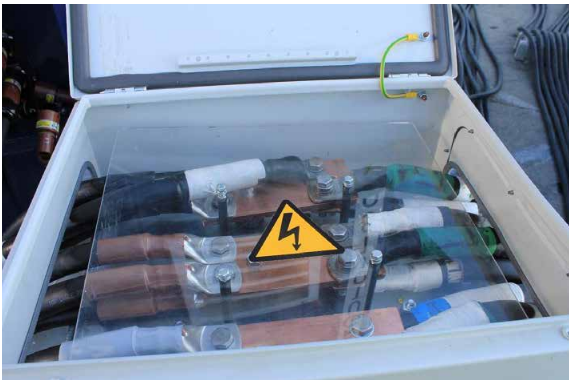
Figura 141. Junction box (3 phases).
