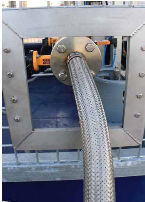
Figura 75. Connecting the gas hose to the tank container.
