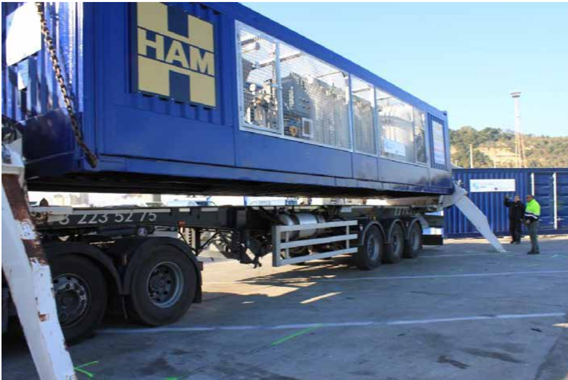
Figura 18. Unloading the container of the LNG tanks at the agreed site.
