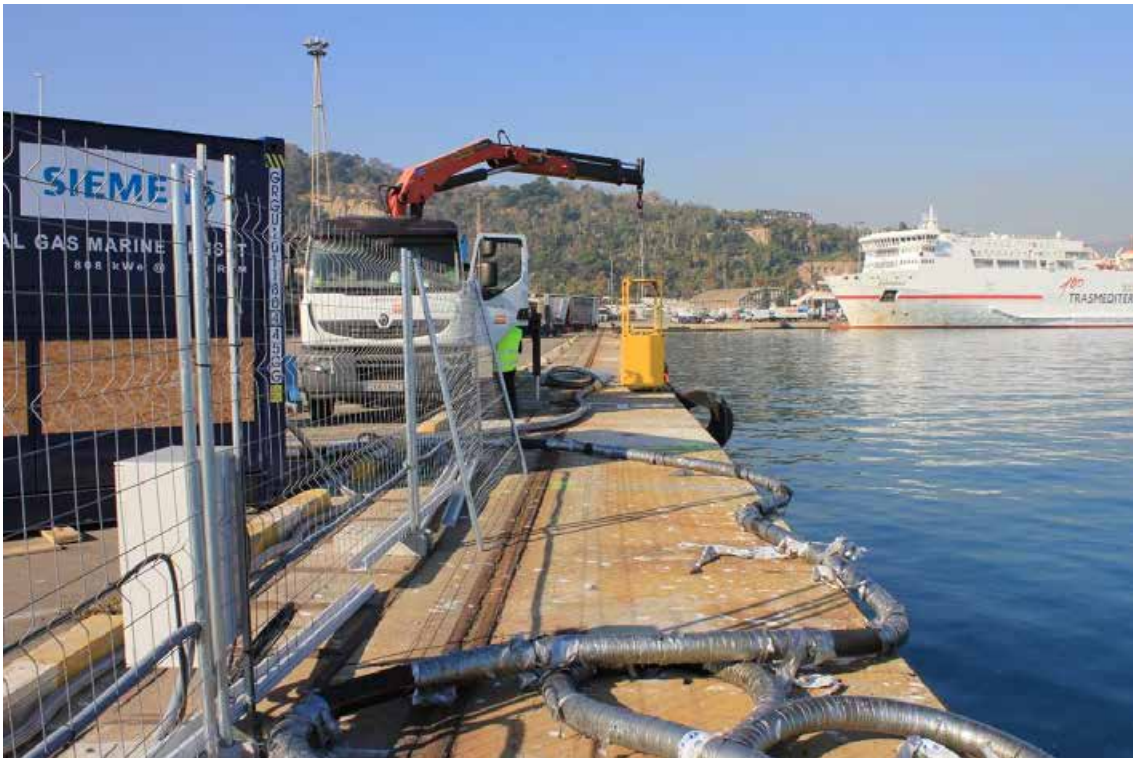
Figura 61. Crane with the cage to access the wharf edge.
